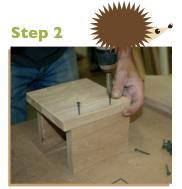
Drill and countersink the top of the 'tunnel' to the sides, then secure with galvanised screws.
